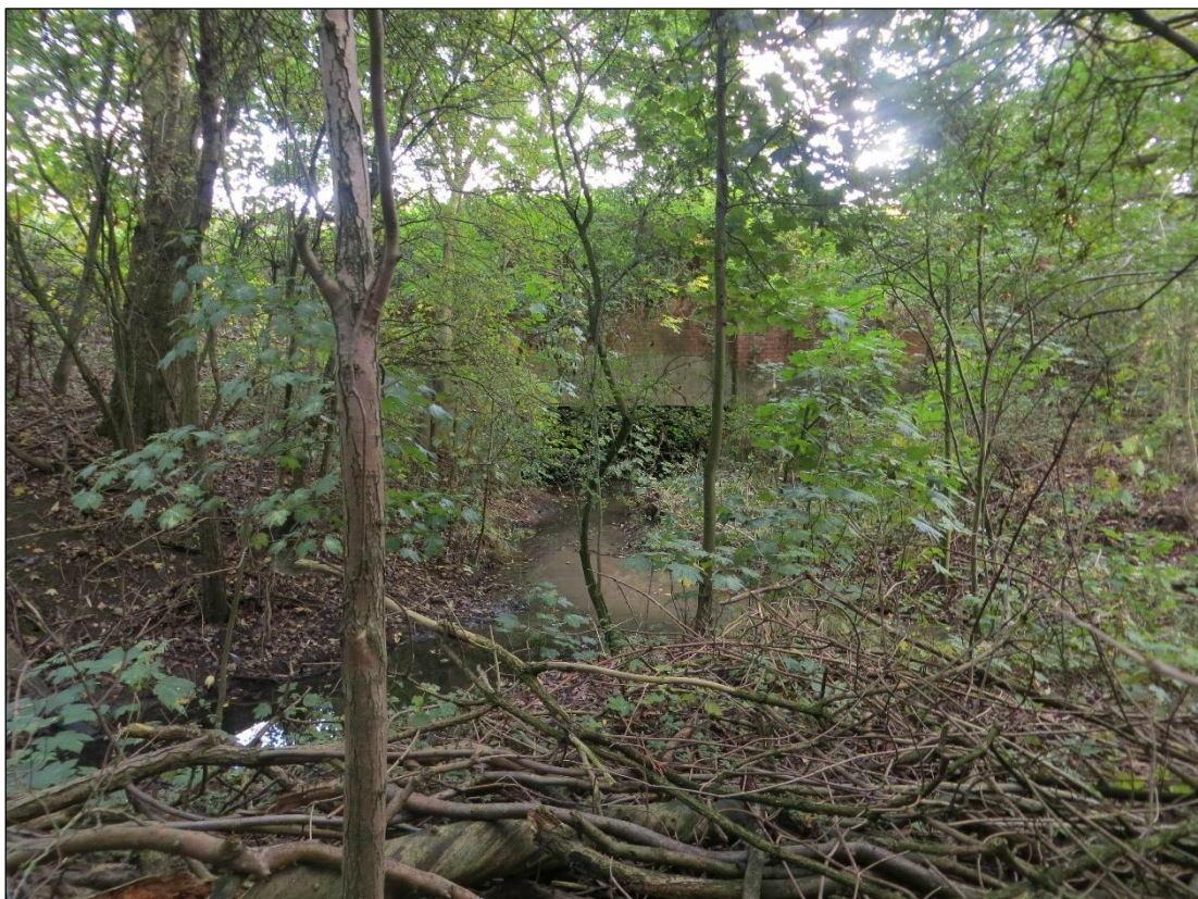
Figure 5.3 – Courteenhall Brook flowing into M1 Culvert
